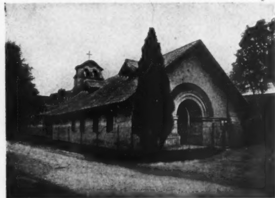
CHURCH IN WONERSH, ENGLAND MR. C. H. TOWNSEND, ARCHITECT
